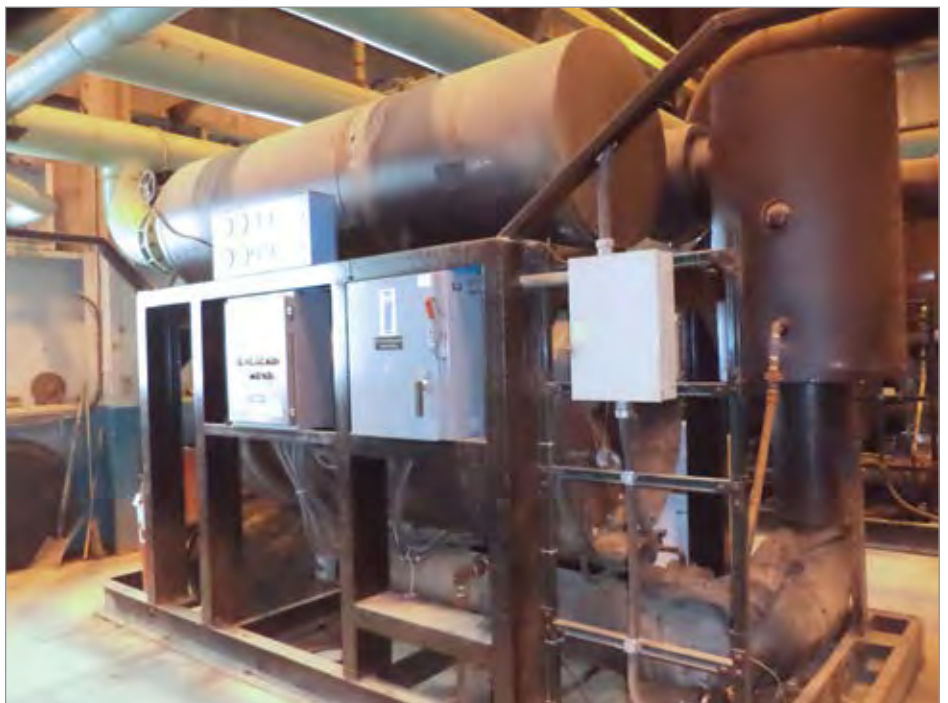
Figure 3: Hybrid-style dryers are used onsite to condition the air for the smelter. This is the 10,000 cfm rated refrigerated part of the combined refrigerated/heated/blower desiccant unit.
