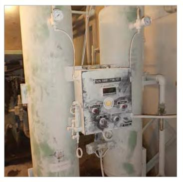
Figure 4: When maintenance and general housekeeping is lacking, the controls can easily fail.
