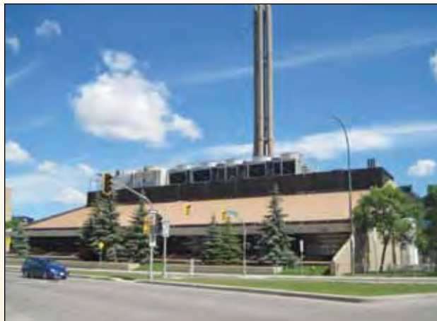
Health Sciences Centre — Central Energy Plant
