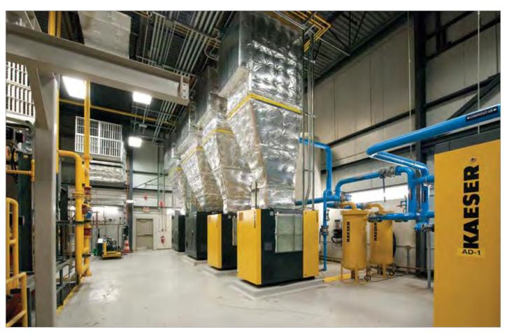
Heat from the new air compressors is recovered in the compressor area.
