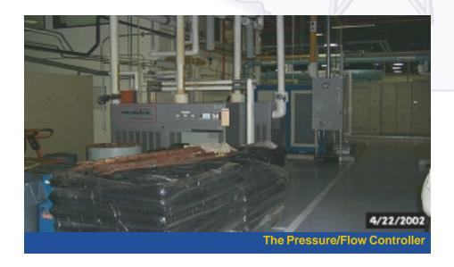
the new configuration, the increased storage provides enough air for the end uses to continue operating through demand spikes. As a result, only one compressor is needed to adequately supply the plant's compressed air demand. The plant's average total flow has decreased from 400 scfm before the project to 325 scfm currently. This decrease has been made possible by the leak repair campaign and application of zero loss air drains and solenoid valves that have sharply reduced artificial demand.
